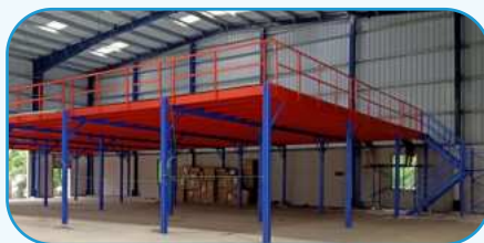
Modular Mezzanine Floor
